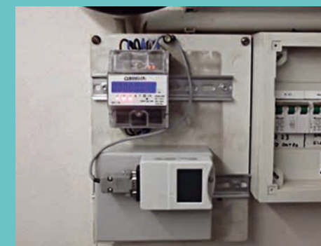
Datalogger S7021 reads and records data from electrometer.
